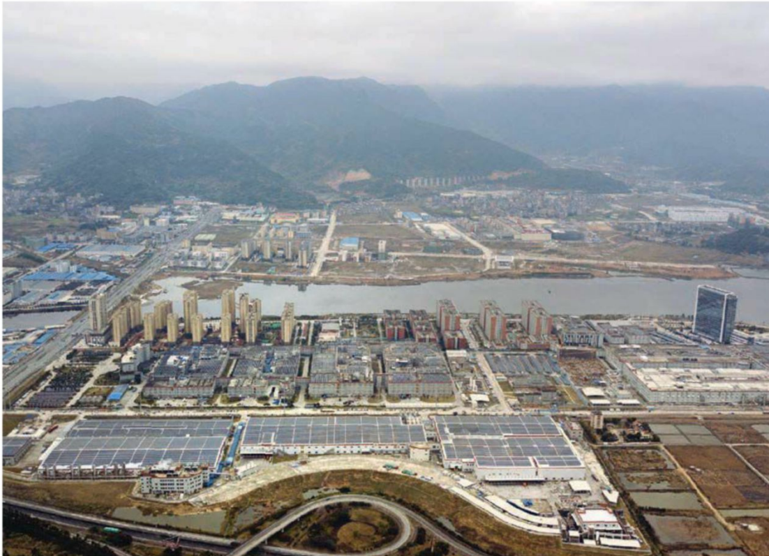
◀ The CATL plant is rising on landfilled mudflats in Ningde, in eastern China
